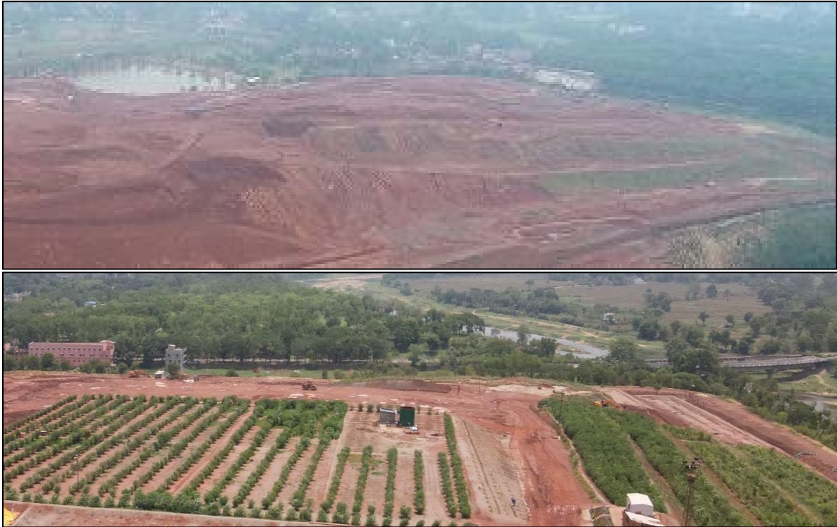
Figure 8. Red to Green :25 acres of red mud yard converted into to green cover in Muri Refinery
